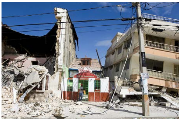
Damaged buildings in Port-au-Prince
